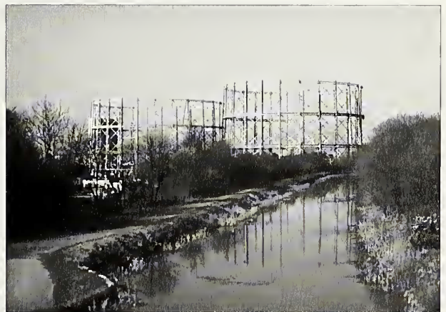
Fig. 1. The structure of the outer cages to the two gasometers at Temple in Glasgow offers many convenient niches where a pair of ravens could build a nest.
